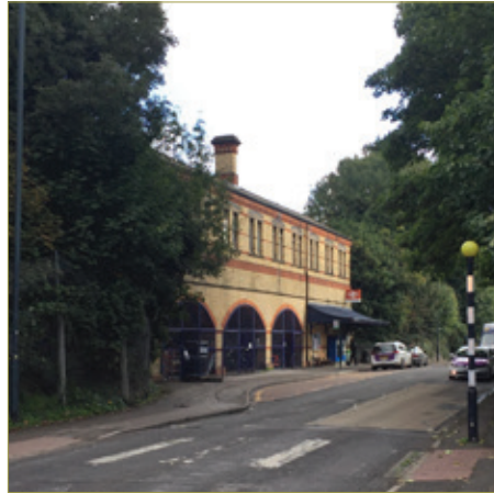
Maidenhead Railway Station access off Shoppenhangers Road
